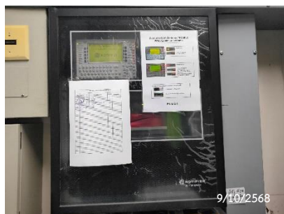
Fire Alarm Control Panel
