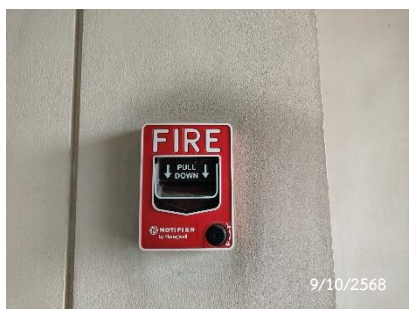
Fire Alarm Manual Station
